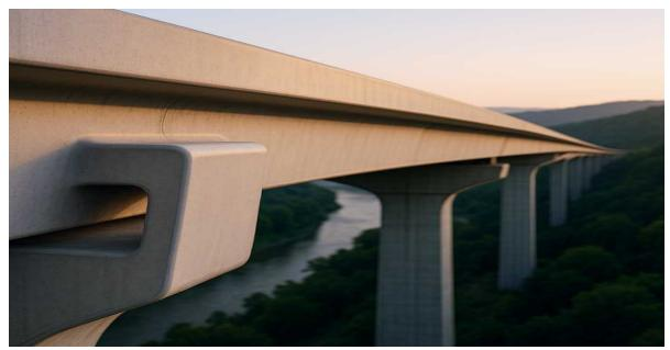
Silane sealing on bridge decks prevents chloride ingress and freeze—thaw damage, preserving rebar and extending deck life.
