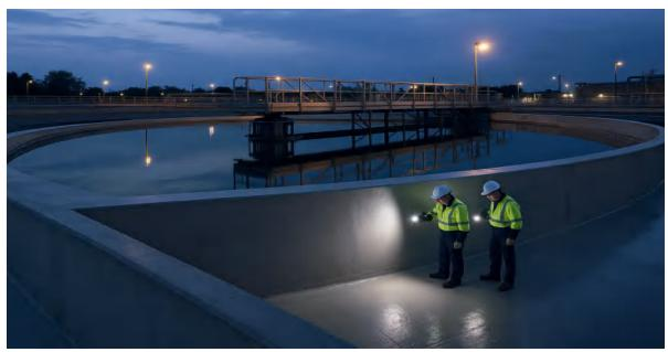
In treatment plants and tanks, silane impregnation blocks chemical attack and moisture ingress, ensuring long-term watertightness.
