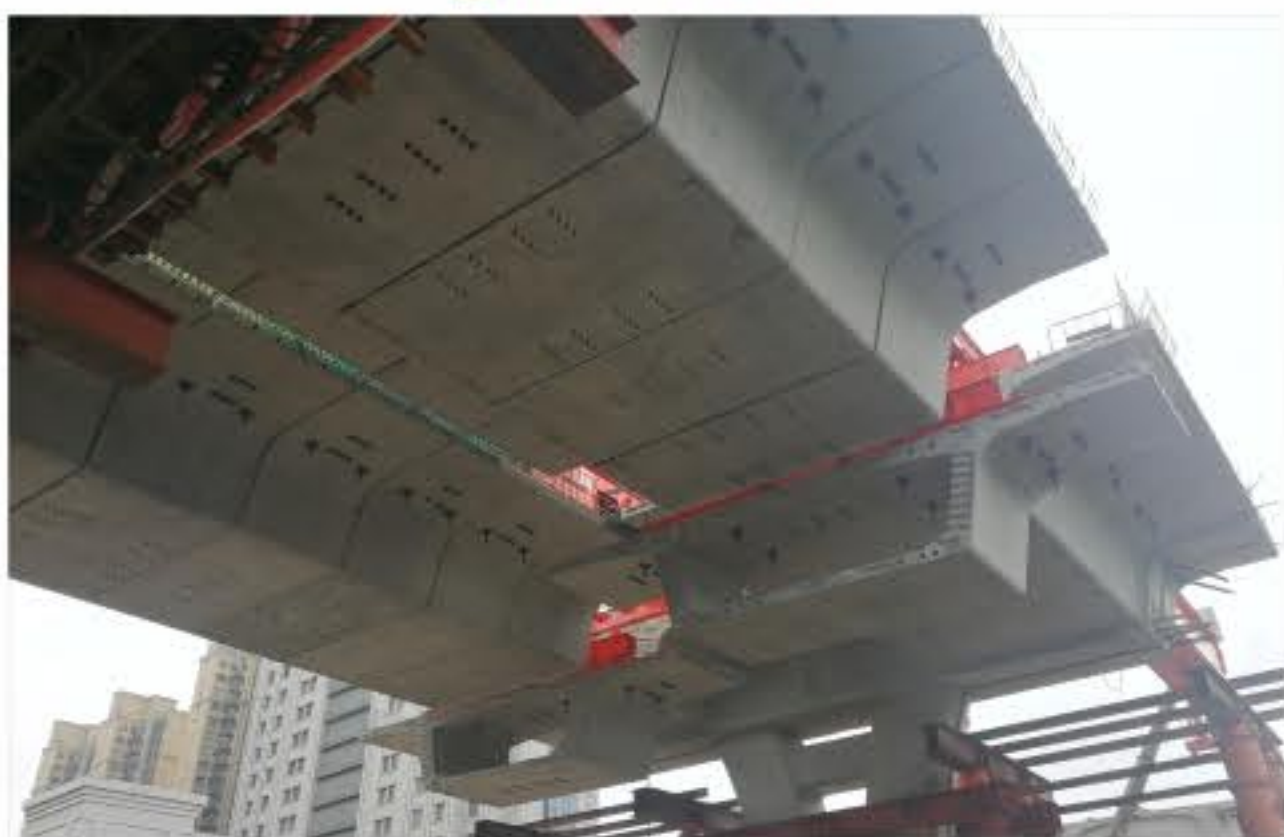
Application of UHPC in precast girder box
