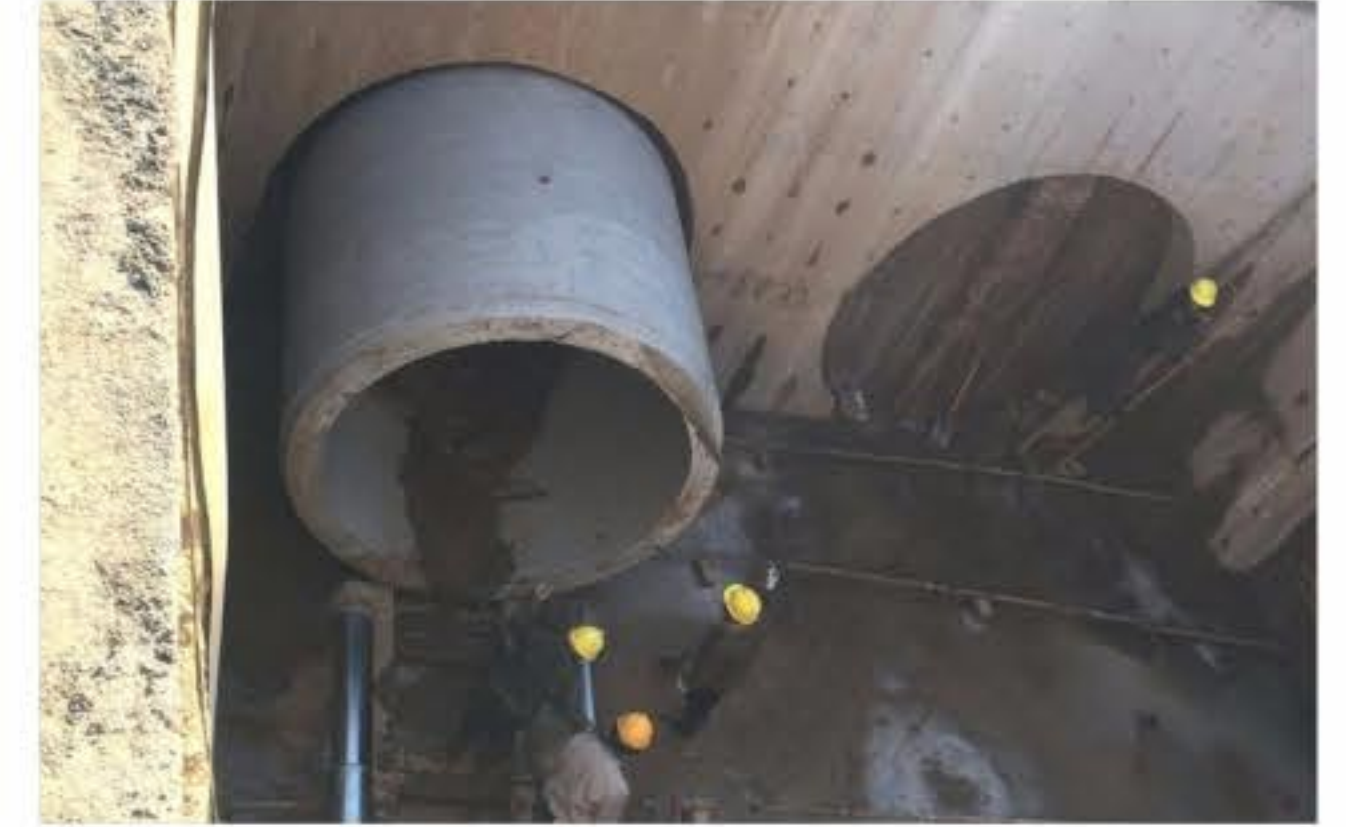
UHPC in sewage pipes
