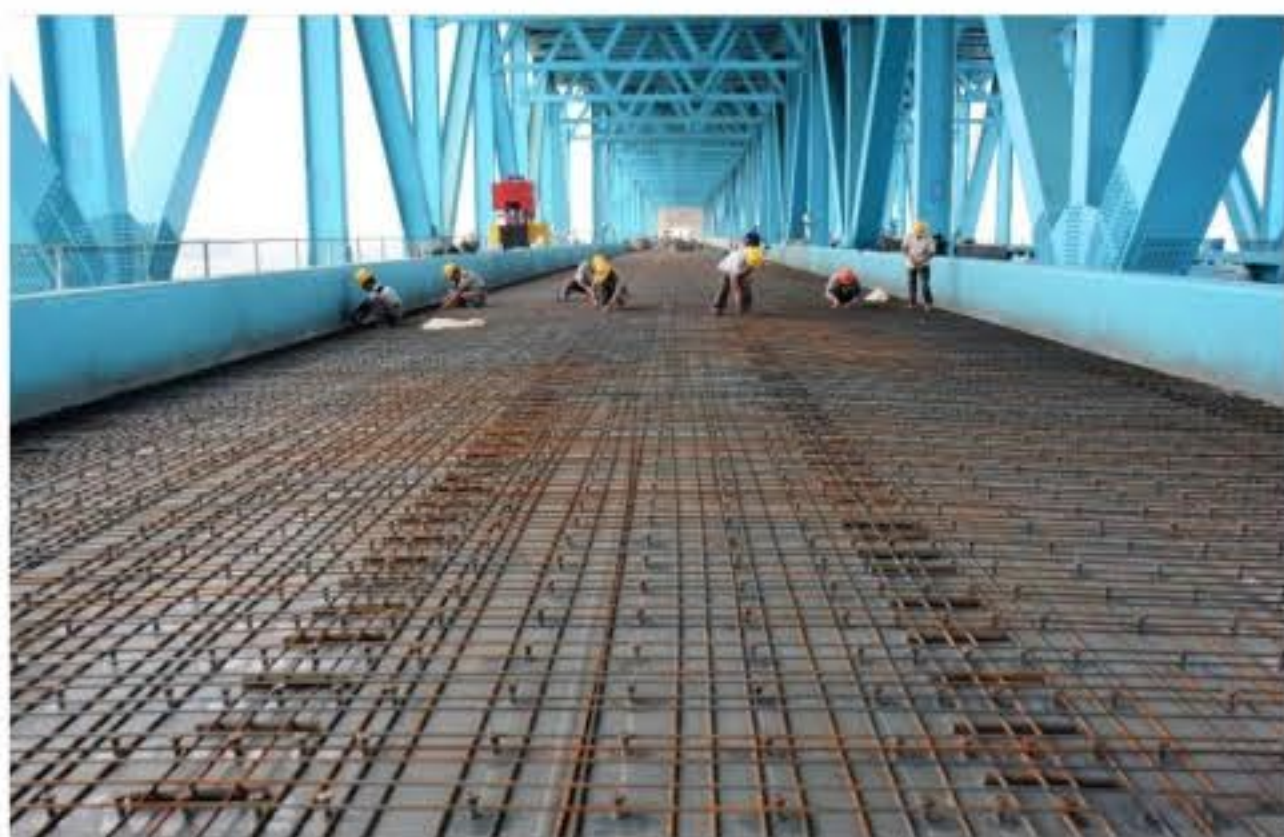
Application of UHPC in bridge paving
