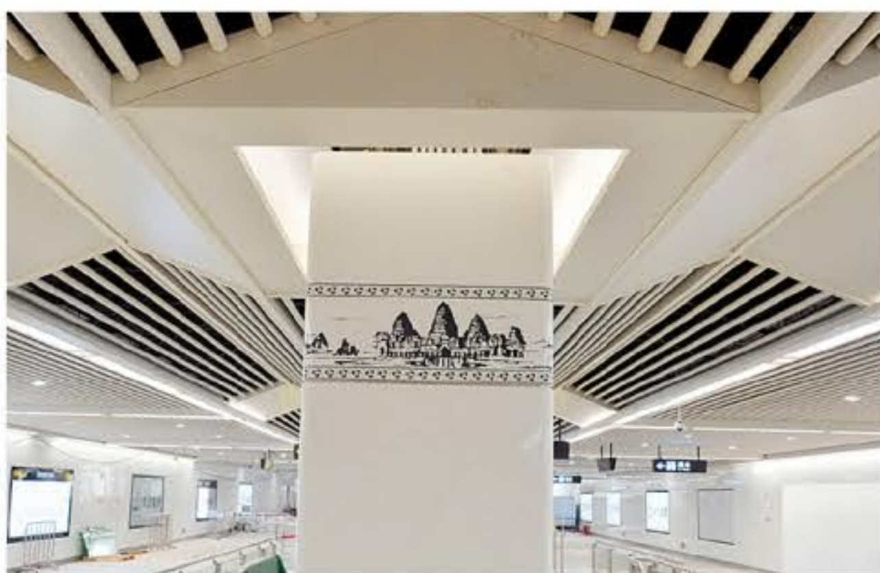
Application of UHPC in underground decorative panels
