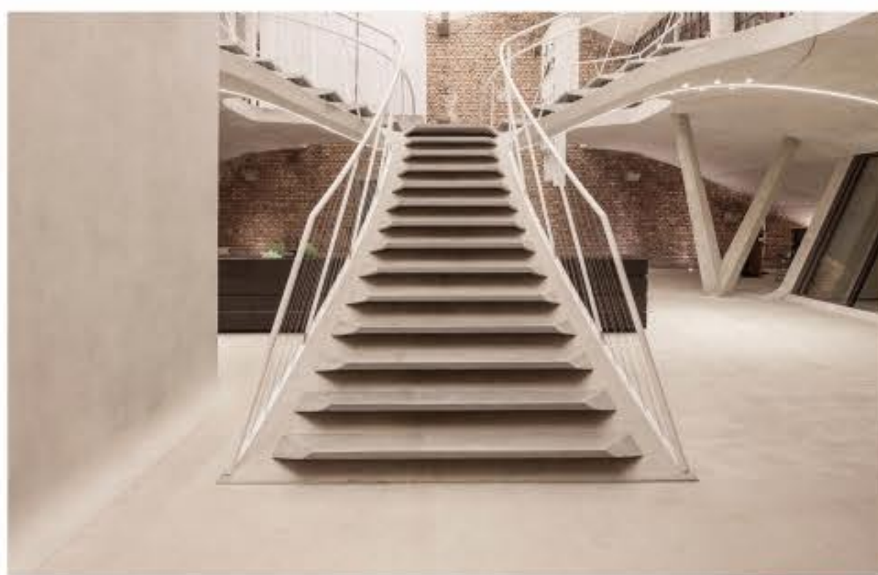
UHPC in lightweight staircases
